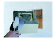
Press the MTH QUADRO PU mounting blocks until they are flush with the insulation panels.
