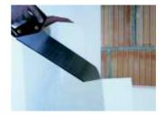
Apply adhesive mortar to the surface of the MTH QUADRO PU mounting block to be attached. The element must be completely covered over the entire surface of the base.
